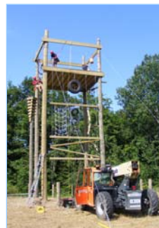
Construction begins on the Above the Falls Challenge Course
